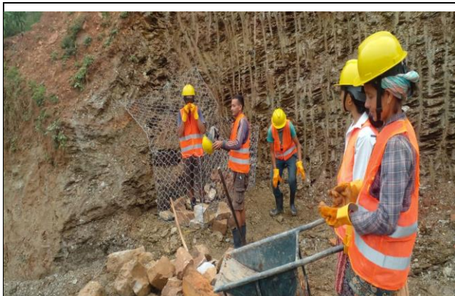
Road under construction- Simta 2
